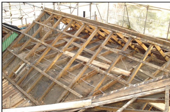
Under the tent the roof rafters are exposed for inspection/replacement
