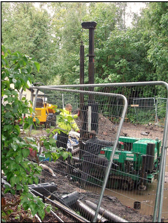
Sinking the piles
