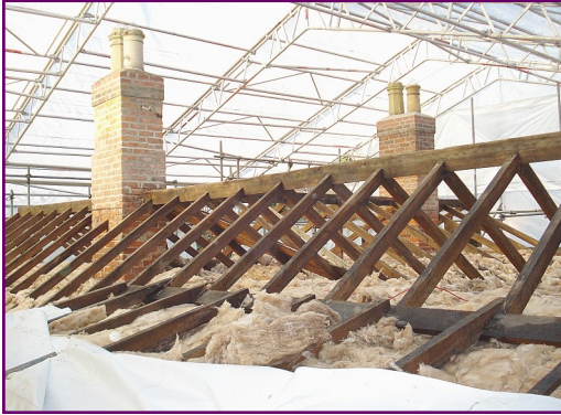
Insulating the Bungalow Roof
